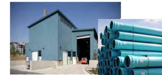
DISTRICT WATER Non-Potable Water System
