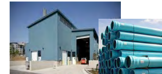
DISTRICT WATER Non-Potable Water System
