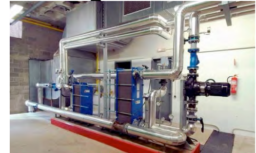
BUILDING CONNECTION Heat Exchanger
